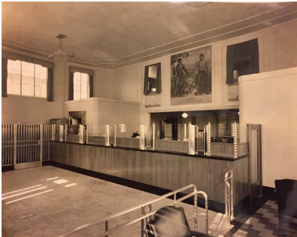
Figure 4.3-3b: Interior of the Village Municipal Building
