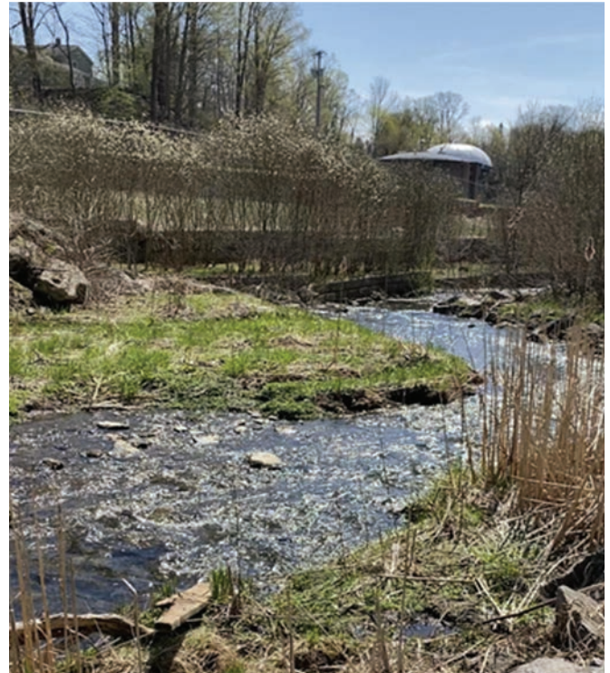
Figure 5.3-4: View of Spring Brook and the Sewage Treatment Plant from Existing Service Trail
